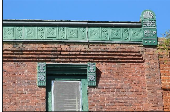
Figures 1 and 2: Cornice features at the top of exterior walls on existing historic buildings.
