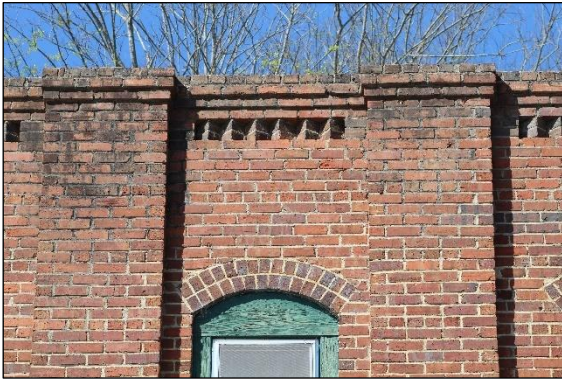
Figures 1 and 2: Cornice features at the top of exterior walls on existing historic buildings.
